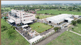
PIX Transmissions Limited MEC Plant
